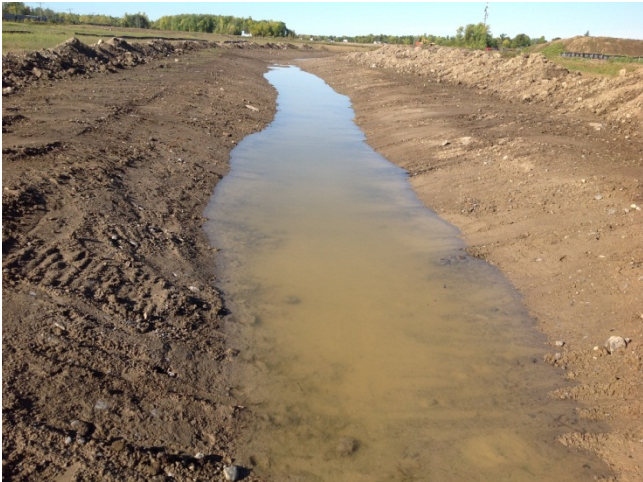
Photo 9: Tributary of Hoople Creek (September 2012) - Facing upstream (west) From Dickinson Drive, showing newly constructed channel, at connection to existing channel will connect.
