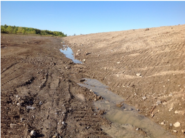
Photo 5: Tributary of Hoople Creek (September 2012) - Facing upstream (west) at middle of property showing realigned channel immediately following construction before vegetation growth.
