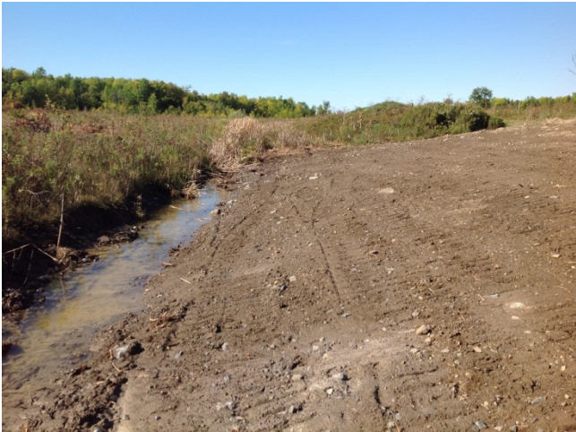
Photo 3: Tributary of Hoople Creek (September 2012) - Facing upstream (west) where existing channel converges with newly constructed channel, immediately following construction before vegetation growth.
